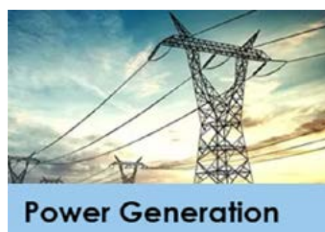
Fig. 3: Electrical power grid fed with power generated from natural gas
